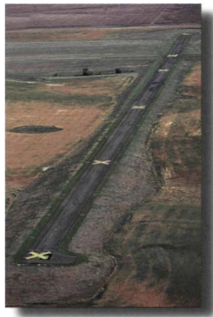
Figure 4-20. Although the surface may appear to be usable, operations on a closed runway cannot be conducted safely.
